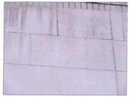
option would be desired, the cracks could be routed and sealed with a new polyurethane sealant; however this option is generally considered unsightly and is not recommended.
