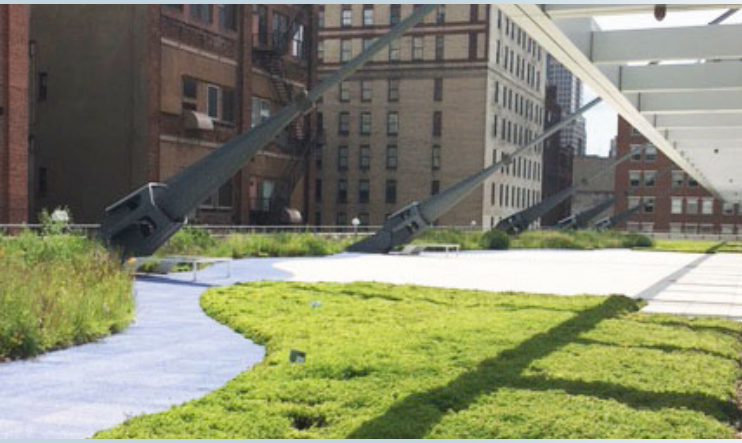
South Terrace Green Roof
