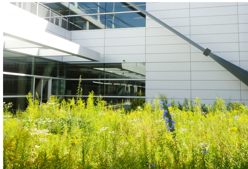
South Terrace Green Roof
