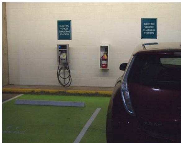
EV Charging Stations in DLCC Garage
