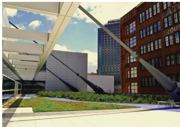
South Terrace Green Roof
